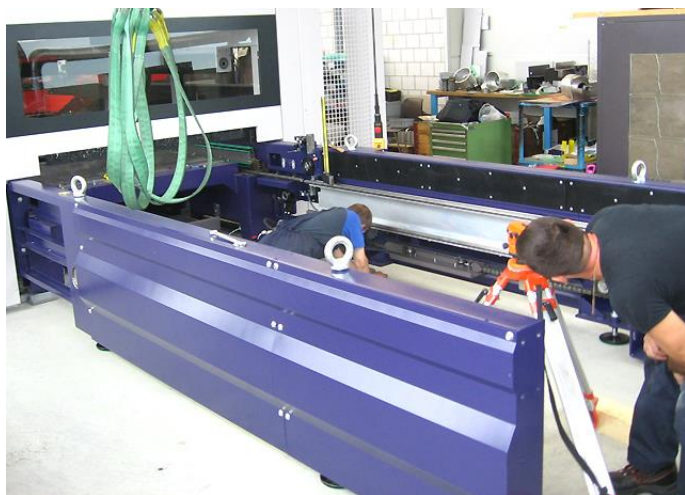
Mounting of laser cutting machine assembly
