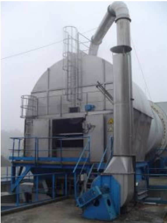
Fermentation pipe View image
