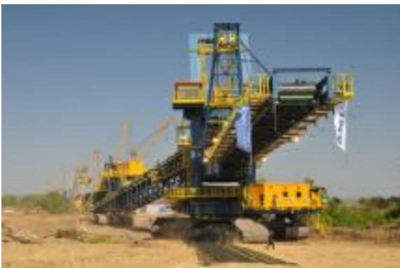
Production and assembly of spreader ARS 2000 with tripper car, TKF, TE Kostolac
